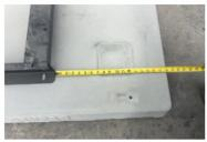
Rather than centering the installation, line up the generator frame so that the GenPad LC's knockout aligns with where conduit will be run. This will leave an apron of approximately 17" at one end.
