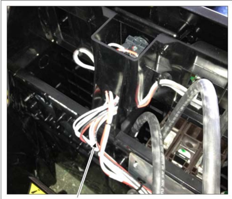
FIGURE 5. ROUTING OF THE EMERGENCY STOP CONTACT BLOCK WIRES (GENERATOR SETS WITH A DISPLAY PANEL KNOCKOUT ONLY)
