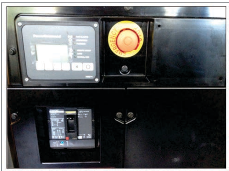
FIGURE 12. INSTALLED EMERGENCY STOP SWITCH KIT (GENERATOR SETS WITH A DISPLAY PANEL KNOCKOUT ONLY)
