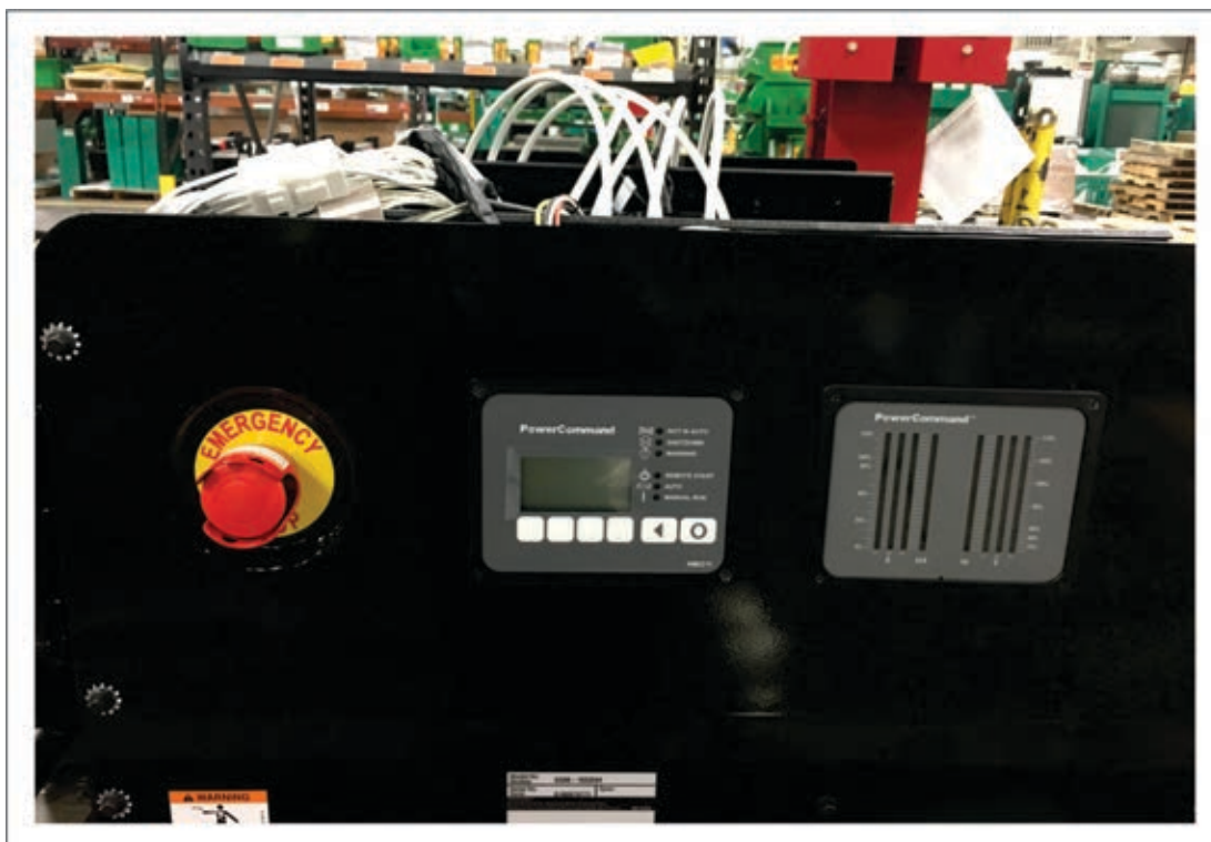
FIGURE 13. INSTALLED EMERGENCY STOP SWITCH KIT (GENERATOR SETS WITH A DISPLAY PANEL RUBBER PLUG ONLY)
