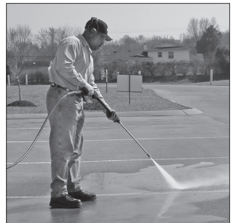
Figure 21 - Optimum angle to cleaning surface
