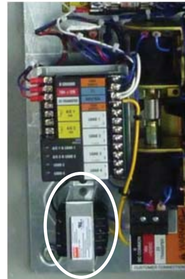
RTSY TRANSFORMER MOUNTING
