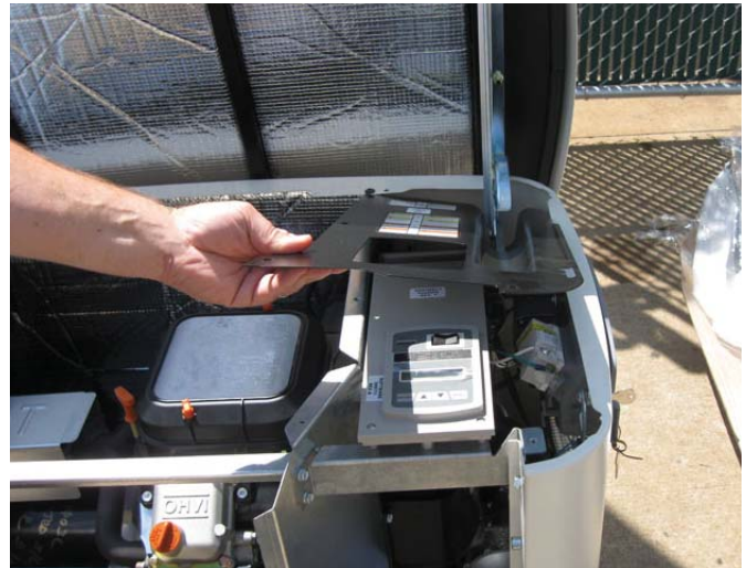
Figure 1 — Remove Control Panel Cover
