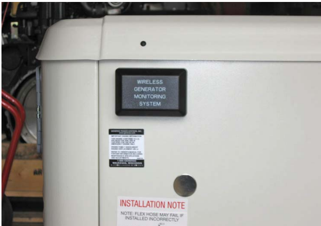
Figure 3 — Mount Transceiver
