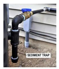
Figure 5.3 — Sediment Trap
