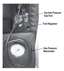
Figure 5.5 — Checking Pressure with Manometer
