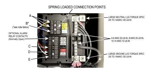
Figure 6.1 — Control Wiring (found behind control board)
