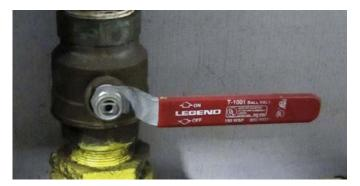
Figure 5.2 — Full Flow Shutoff Valve
