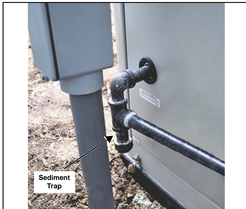
Figure 5-3. Sediment Trap
